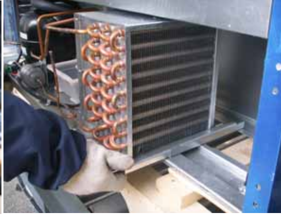
Pull out the condensing unit
